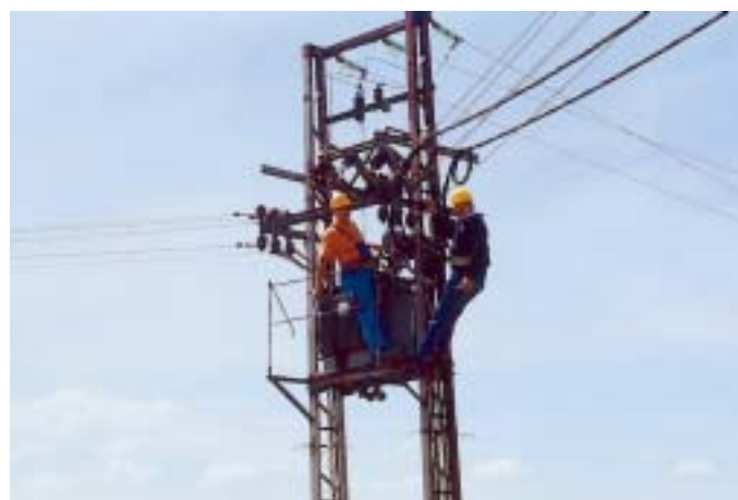
Na TS Galge 2 predradnik Vlado Turković i VKV monter Željko Neralić spajaju novi SKS kabel
