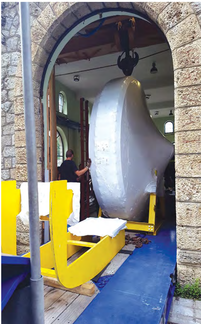
↑ Rotor ulazi u strojarnicu HE Ozalj 1
